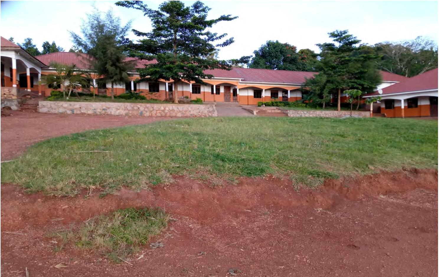
The school is totally rocked down
